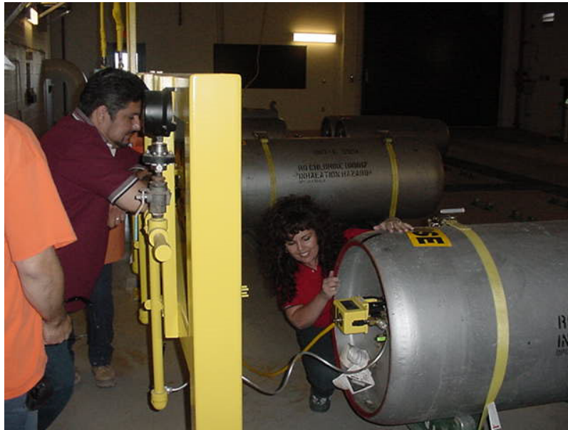
Melissa Durbin showing the proper chlorine gas hook-up procedure. TLC instructors have been to several water providers to show hands-on demonstrations and to teach operators the essentials for providing safe drinking water to the public.
